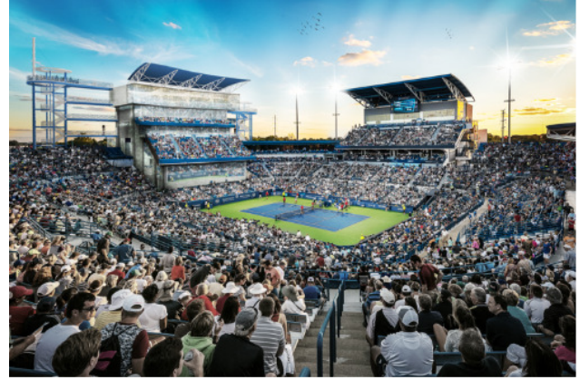
Known as the tennis stadium's South Building, the 40,000 square feet addition 104 foot tall adding significant capability to the tennis facilities. It will open for the 2018 tournament.
