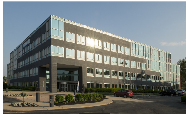
The Mason Tech Elevator, has three locations, 5412 Courseview Drive shown above, the most recent location addition. The 85,000 square foot facility represents the City's P3 initiative to grow entrepreneurial tech and bio companies and is now home to 13 companies and well over 100 jobs.
