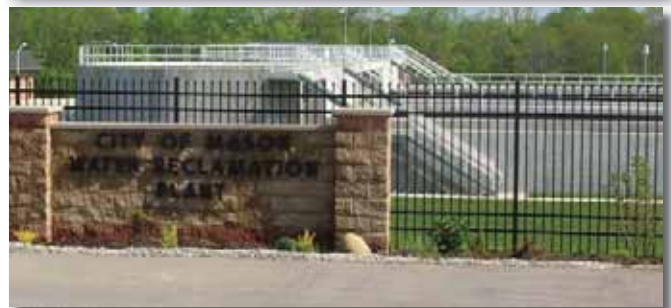
An aerial and street level view of Maon's Water Reclamation Plant located on Mason-Morrow-Millgrove Road.
