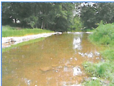
Bank Stabilized with J-Hook Vane and Native Vegetation
